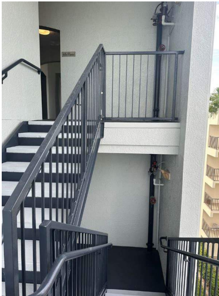
Figure 7: Stairwell, Between 3 rd and 4 th Floors
