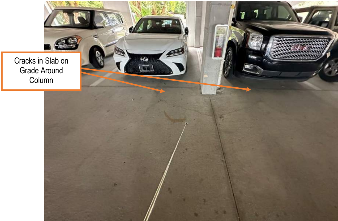
Figure 11: Parking Garage, Ground Level
