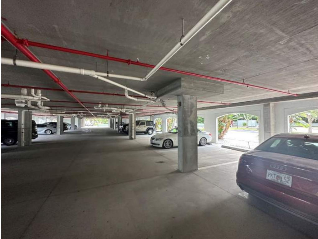
Figure 10: Parking Garage, Ground Level
