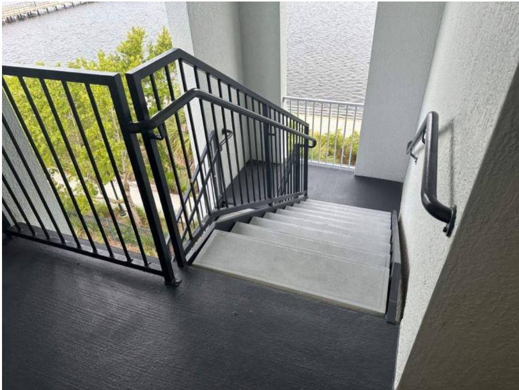
Figure 8: Stairwell, 4 th Floor
